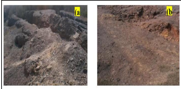
Figure 9: (a), (b), are the field photograph of the year 2015 showing secondary fracture, cracks, fissures/fire etc corresponding to SP anomalies SPAH1/ , SPBH1/ , corresponding to Fig. 8 a.b of profiles AA/ , BB/ respectively.
